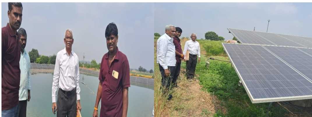
Photo: Farm pond and solar-operated pump in Medsinga village
